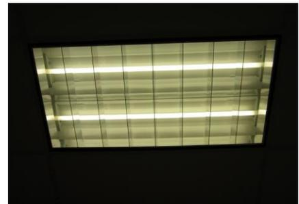
**Figure 2-7:** Two-Lamp, T8 Fluorescent Parabolic Lighting Fixture
