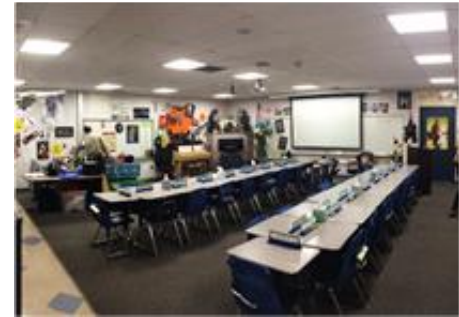
Figure 5: the new lighting system for each classroom includes twelve 2 x 2 recessed, tunable-white LED fixtures. Photo credit: PNNL
