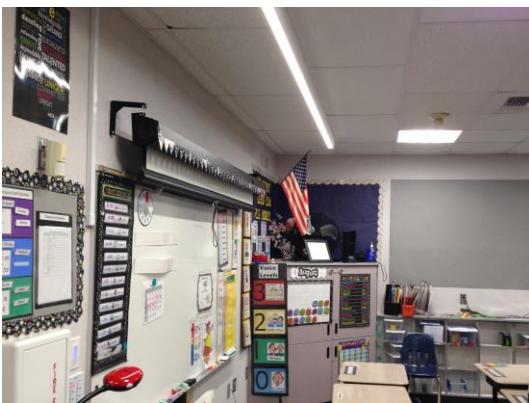
Figure 7: the new classroom lighting systems included wall wash fixtures that could be controlled independently from the recessed fixtures. This feature was especially helpful during presentations.
