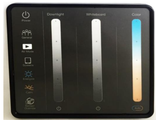
Figure 8: the new classroom lighting systems were controlled by keypads with slider controls and preset lighting scenes. Photo credit: PNNL.
