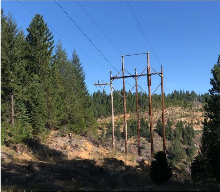
*60kV wood pole design with 4kV attachment*
