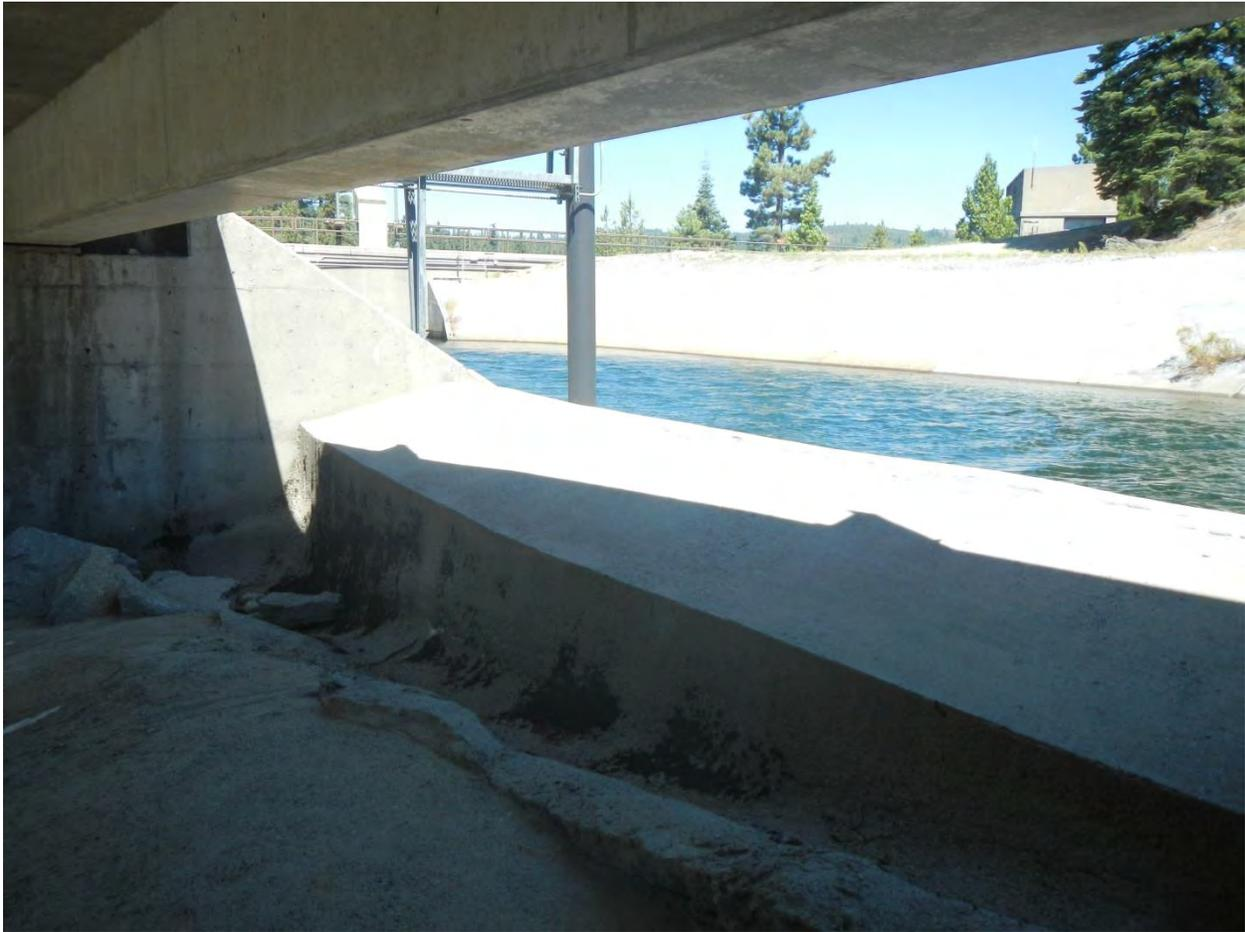
Photo 3. Looking north from below the bridge at the spillway outlet. Note the concrete lining at the outlet.
