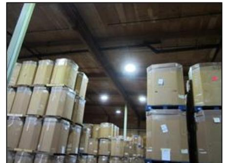
**Figure 4-4: In some locations stacks of boxes blocked the lighting**
