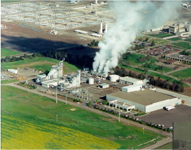
Carson Power Plant
