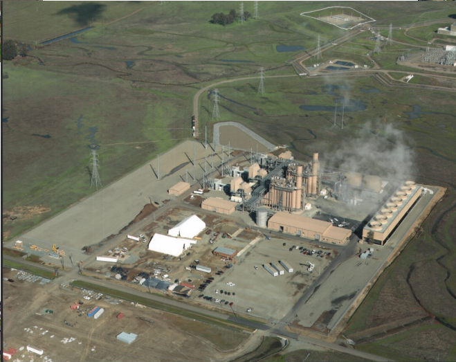
Cosumnes Power Plant
