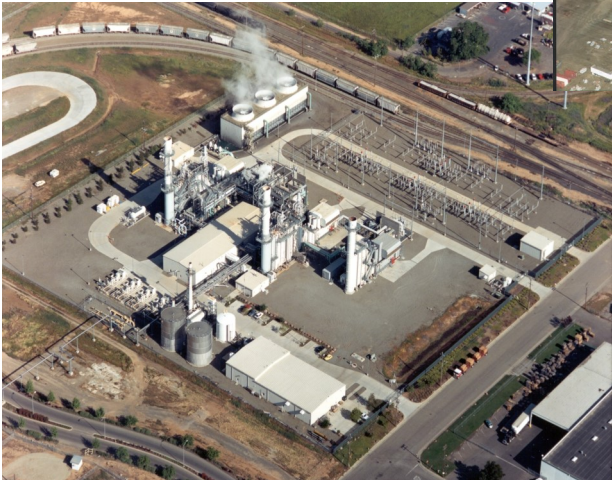
Procter & Gamble Power Plant
