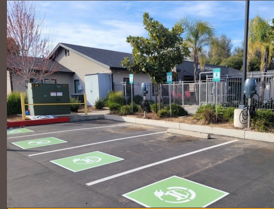
Phoenix Apartments EVSE installation
