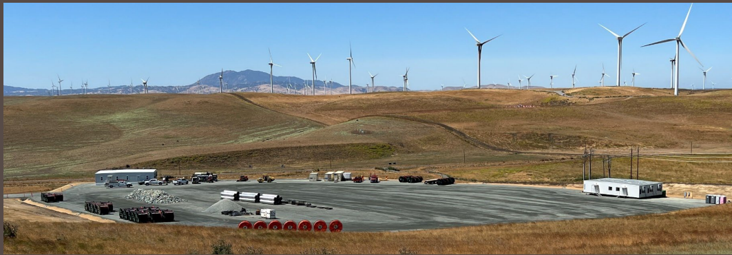
Finish Grading – East Laydown Yard
