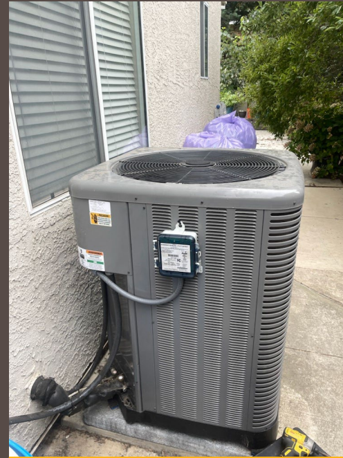
Peak Conserve switch installation
