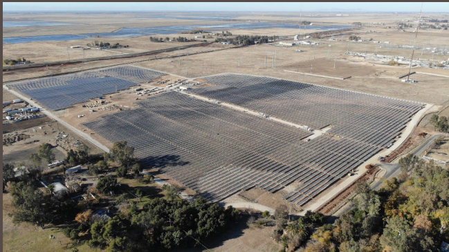
Wildflower PV Array – North Sacramento
