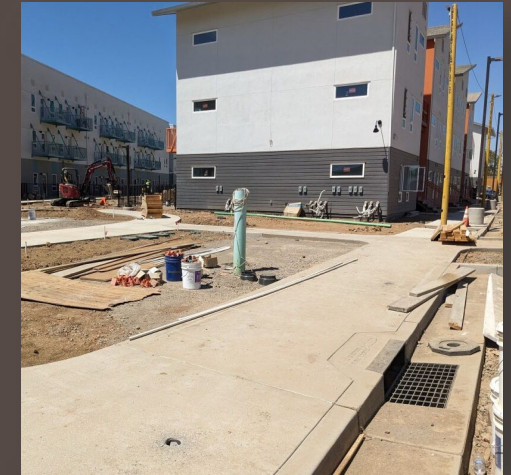
Mutual Housing – “On The Boulevard” multi-family project
