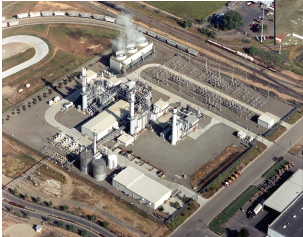
Procter & Gamble Power Plant
