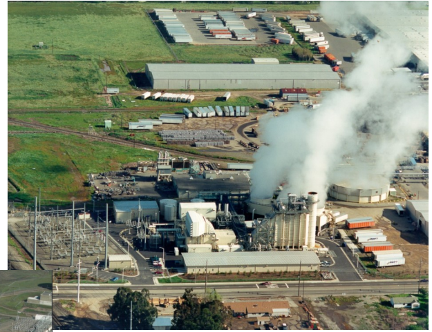
Campbell Power Plant
