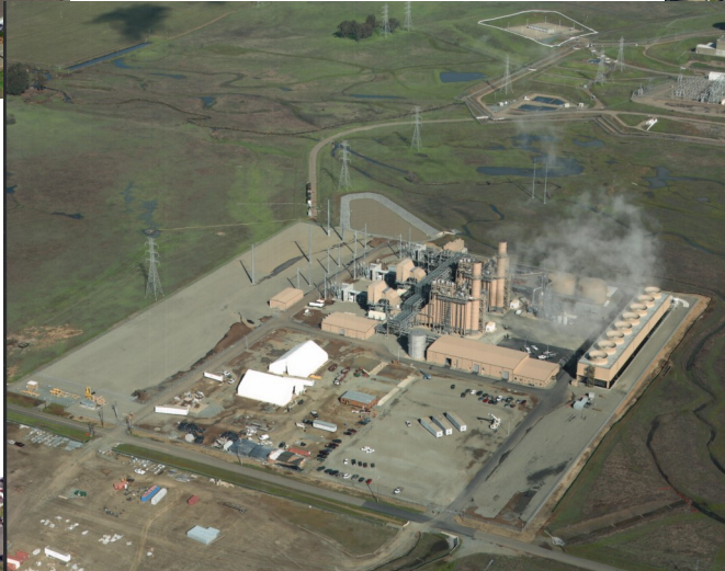
Cosumnes Power Plant
