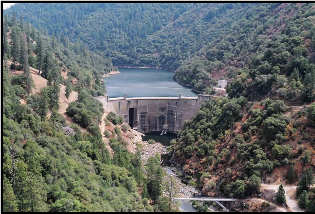
WR-5. Slab Creek Reservoir
