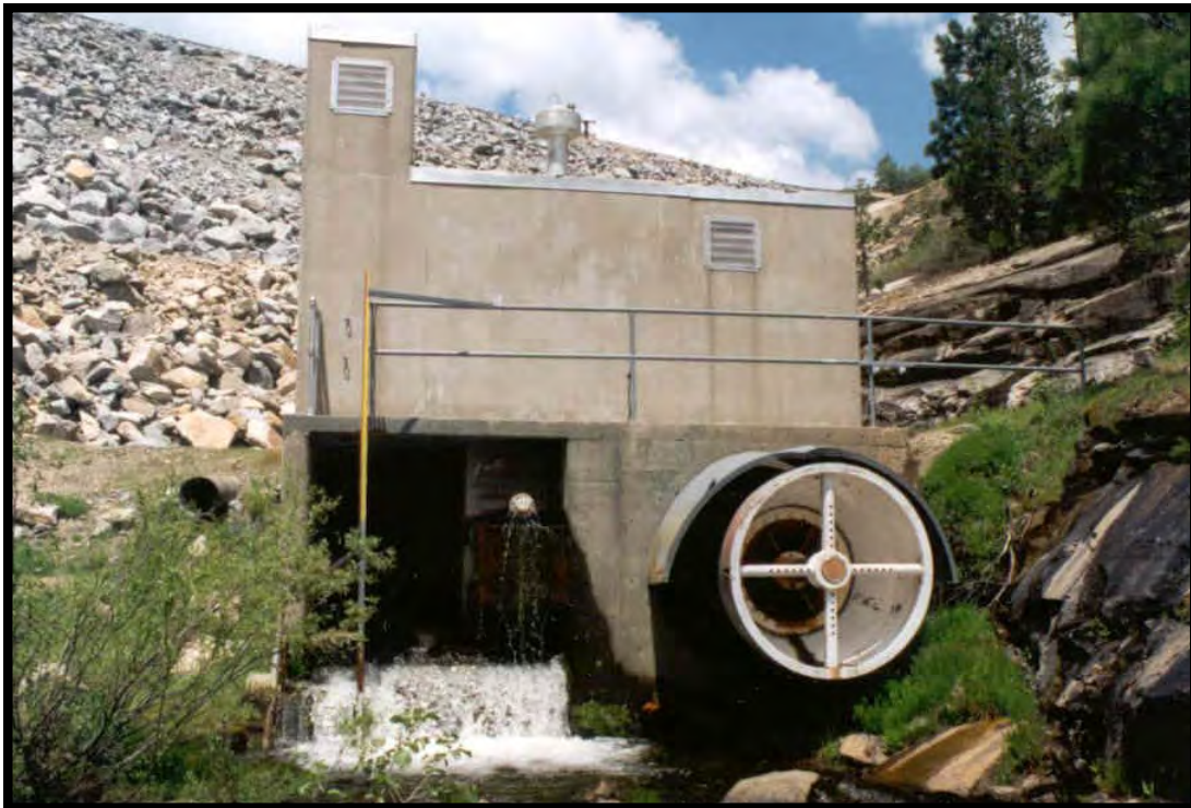
JF-8. Ice House Outlet Structure
