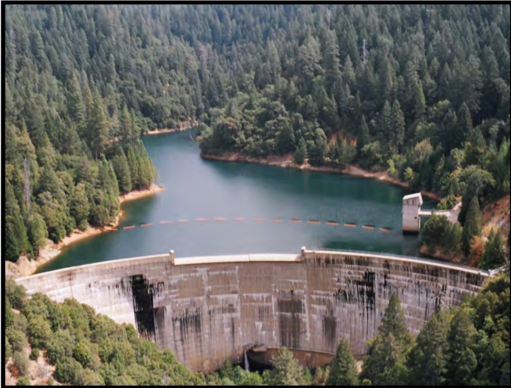
CM-2. Brush Creek Dam and Reservoir
