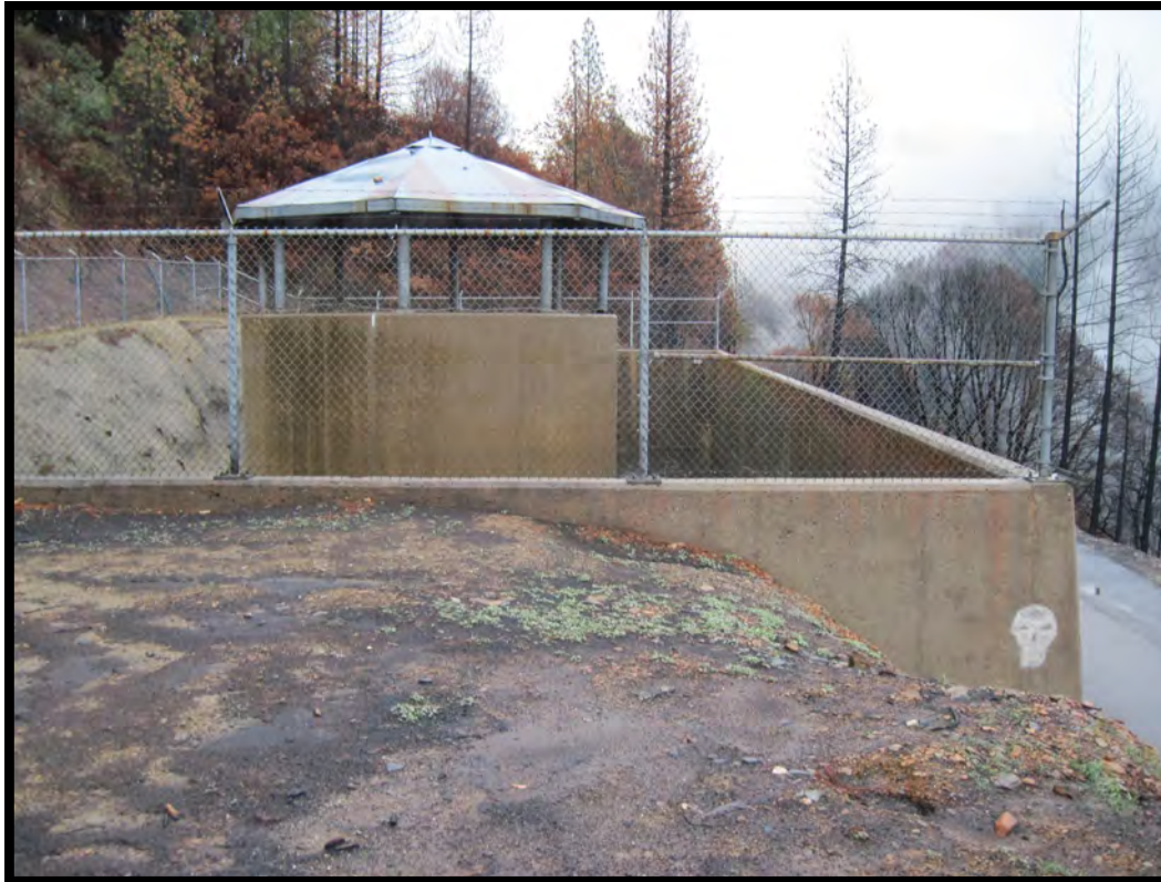
CM-8. Camino Surge Basin
