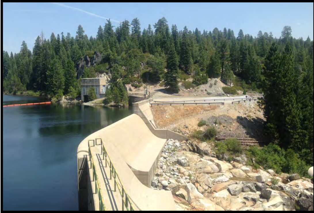
RP-1. Gerle Creek Dam and Loon Tailrace Tunnel Outlet Structure
