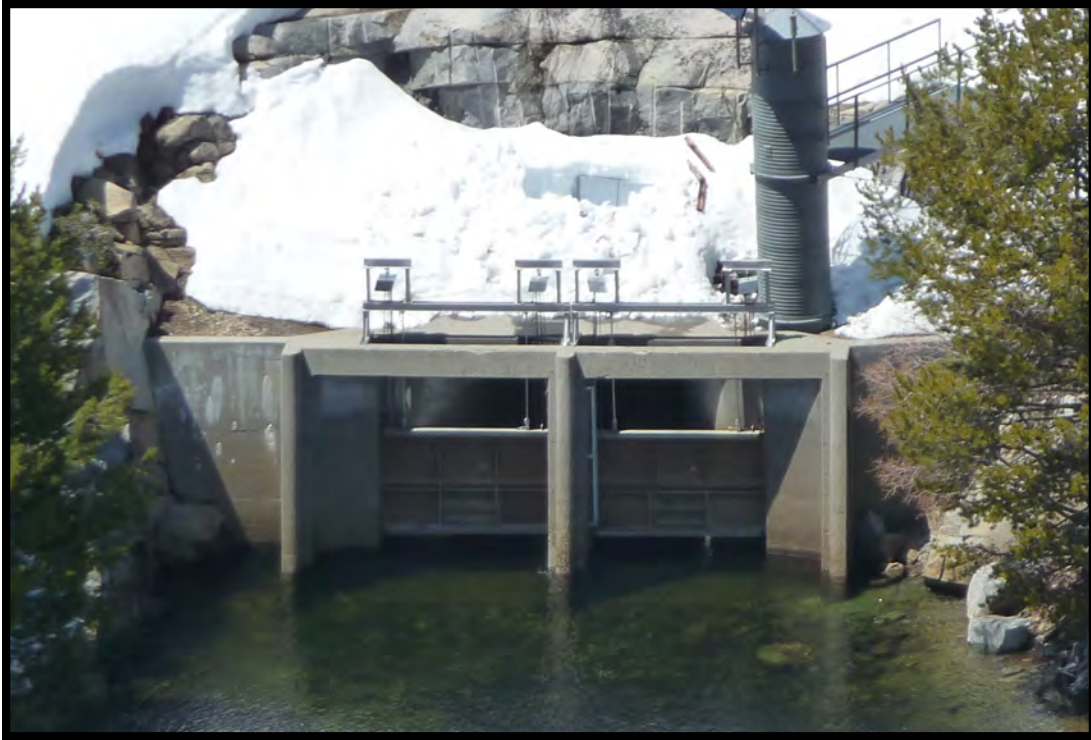
LL-5. Buck-Loon Tunnel Intake
