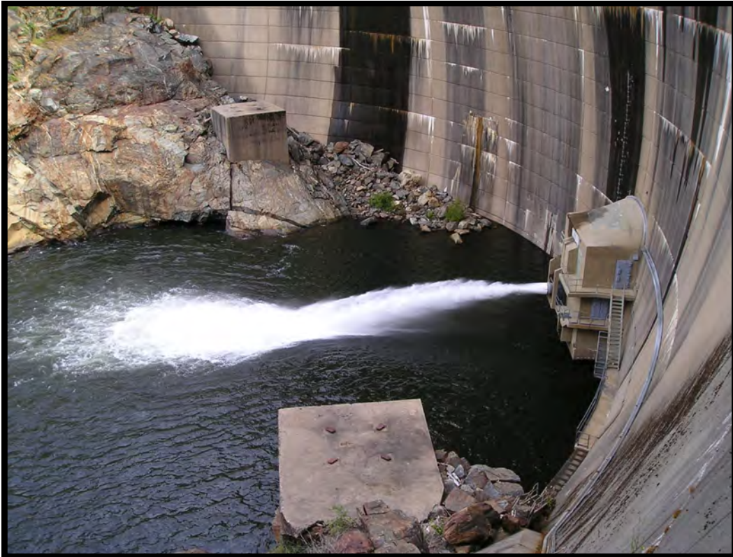
WR-2. Slab Creek Powerhouse and Outlet
