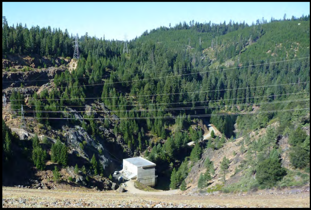
UV-3. Union Valley Powerhouse
