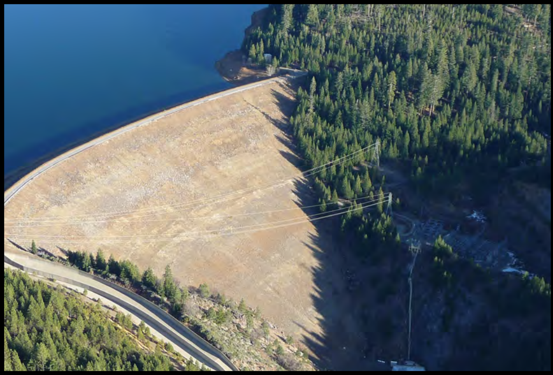
UV-1. Union Valley Dam
