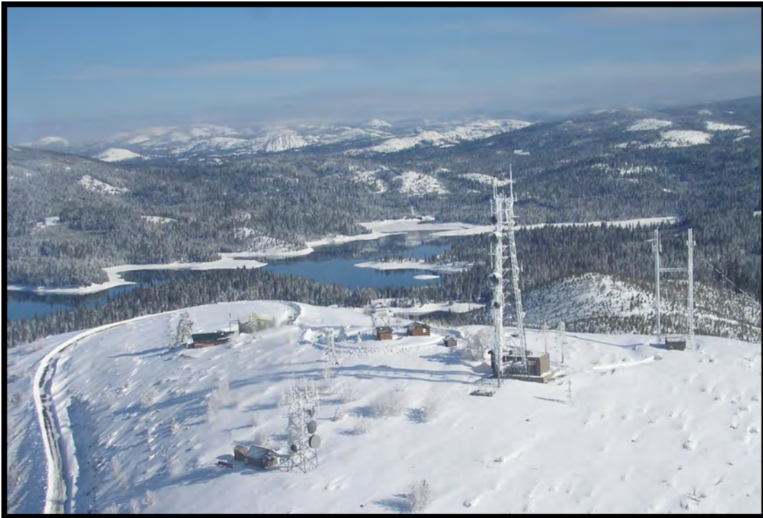
MC-1. Big Hill Telecom Site
