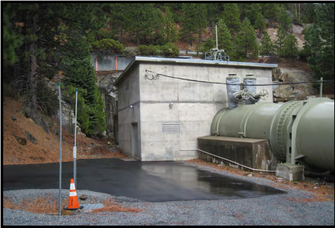
RP-7. Robbs Peak Penstock Valve House
