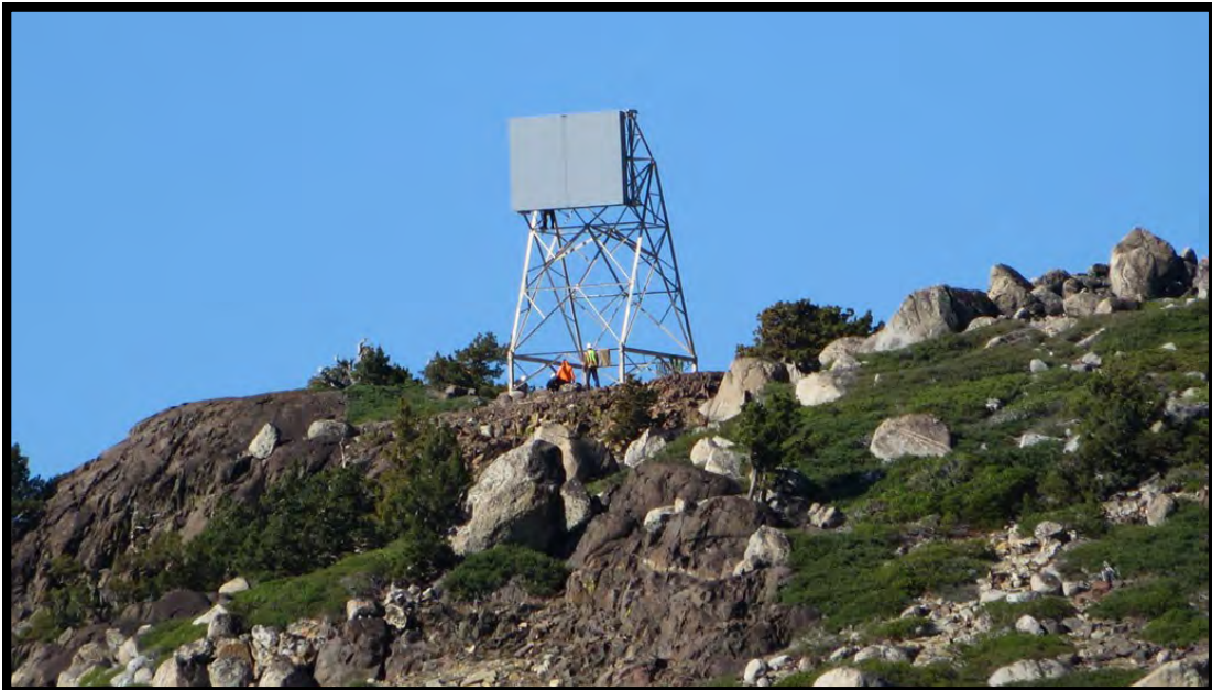
MC-4. Loon Lake Microwave Reflector
