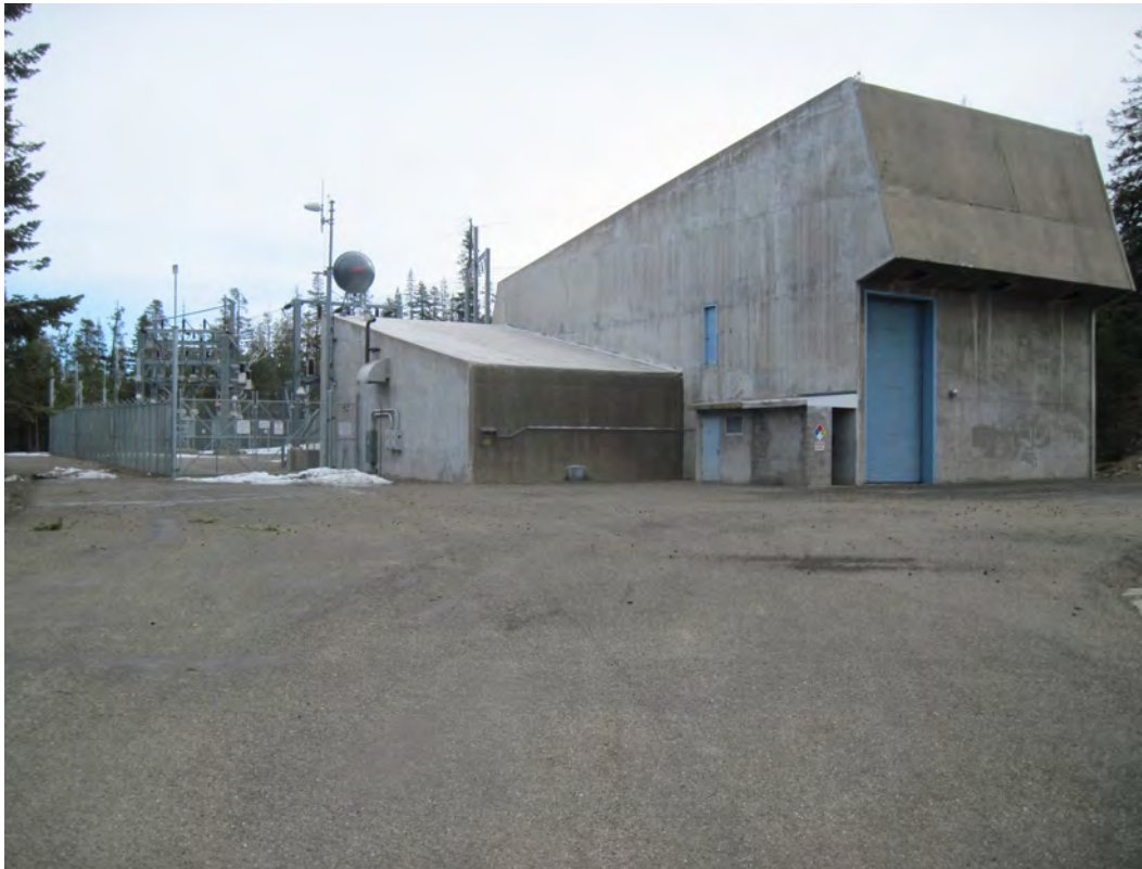
LL-8. Loon Lake Switchyard and Powerhouse Access Building
