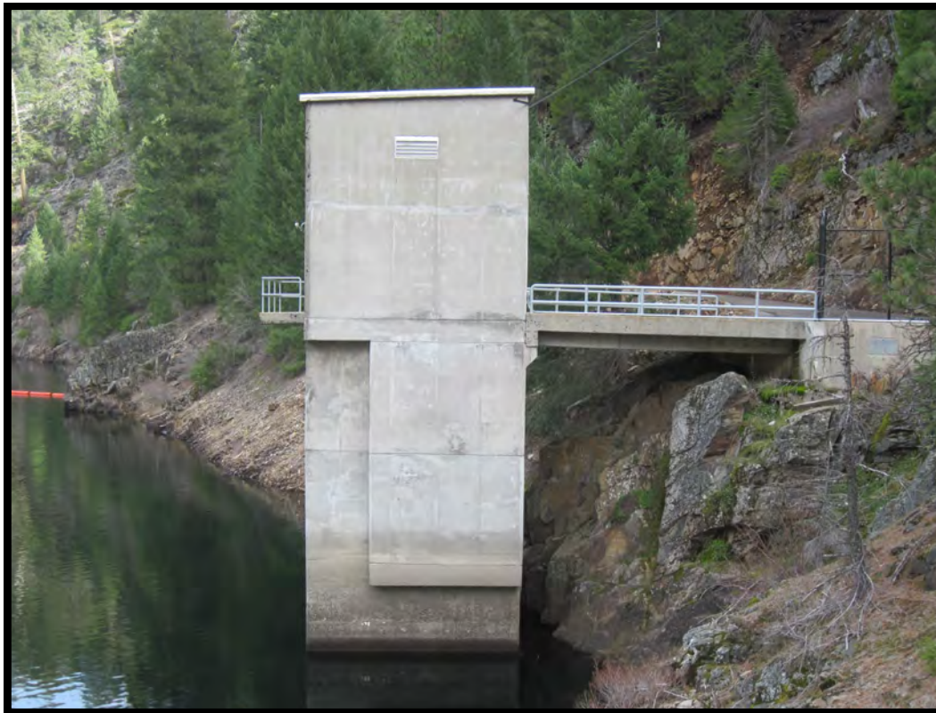
JB-2. Junction Gate House
