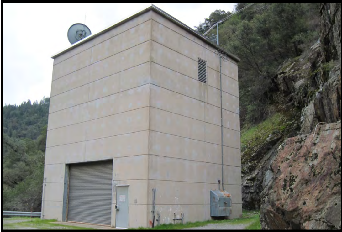
WR-3. Slab Creek Gate House
