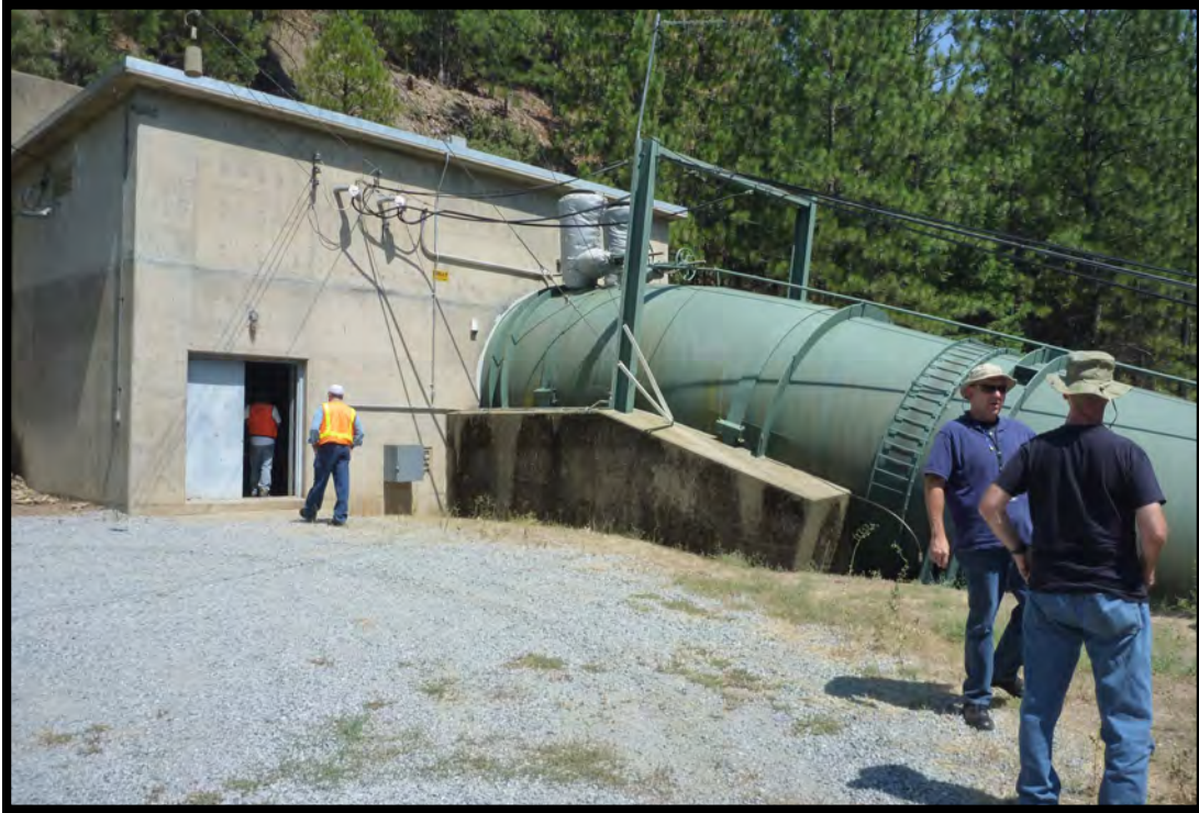
CM-5. Camino Valve House
