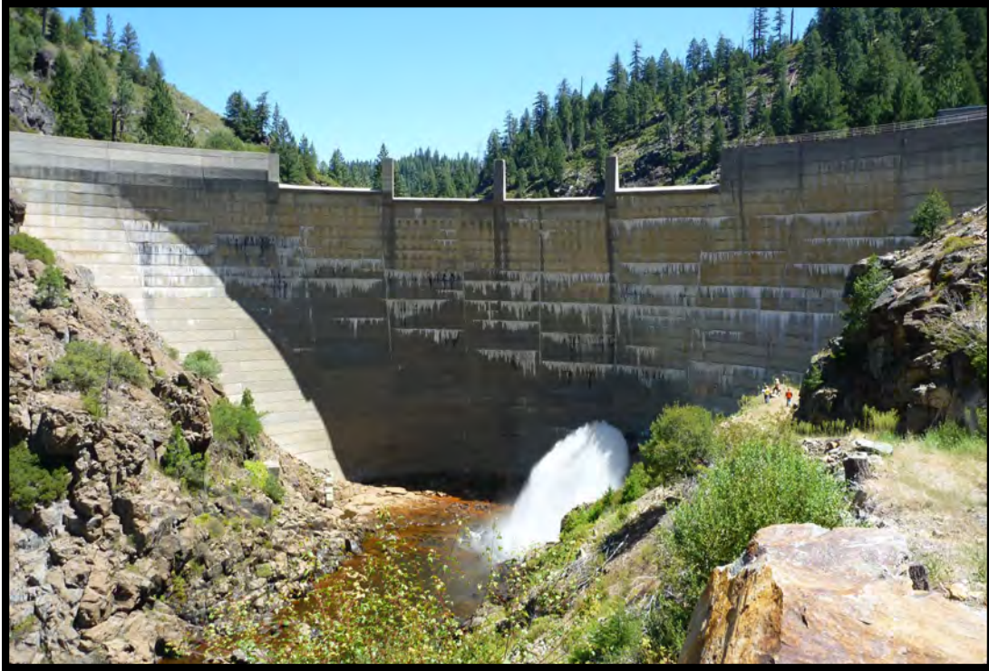
JB-1. Junction Reservoir Dam
