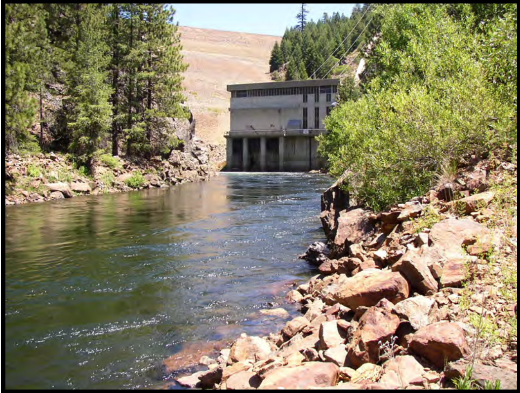
UV-2. Union Valley Powerhouse
