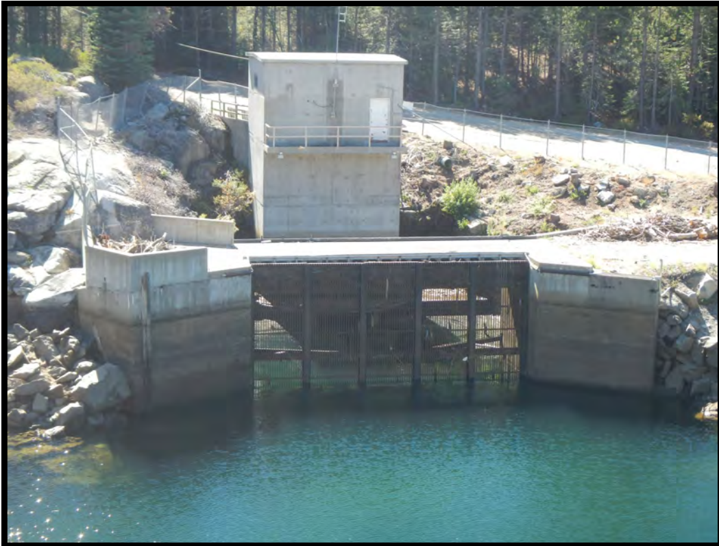
RP-4. Robbs Peak Tunnel Intake/ Gate House
