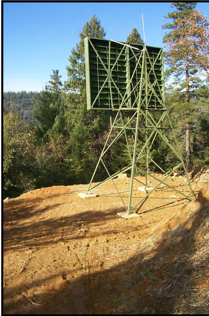
MC-7. Microwave Signal Reflector
