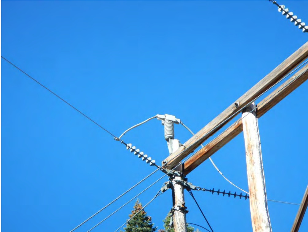
Photo 1. Detail of the insulator product applied to the 69 kV Jones Fork line.
