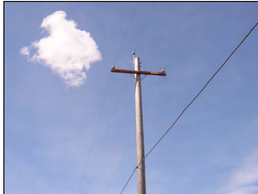
Exhibit 2-5. Small diameter conductors reduce visibility particularly during inclement weather.
