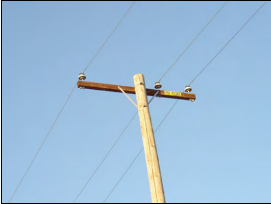
Exhibit 4-14. Three phase, two on one side.
