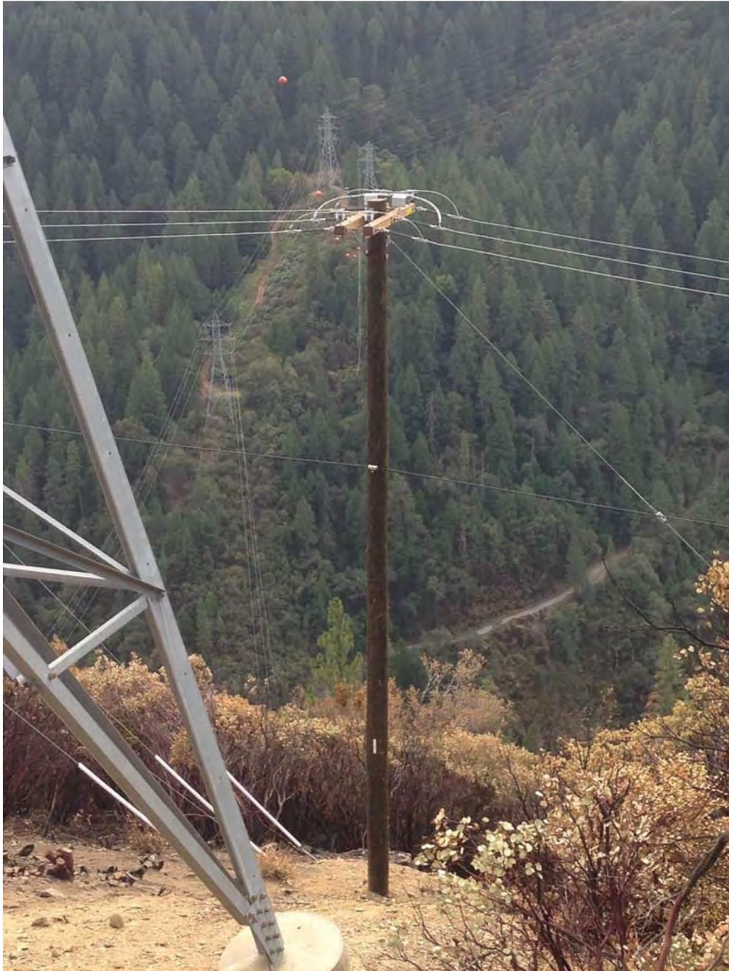
Photo 4. Pole from the rebuilt Brush Creek Tap Line using APLIC-Suggested Practices.
