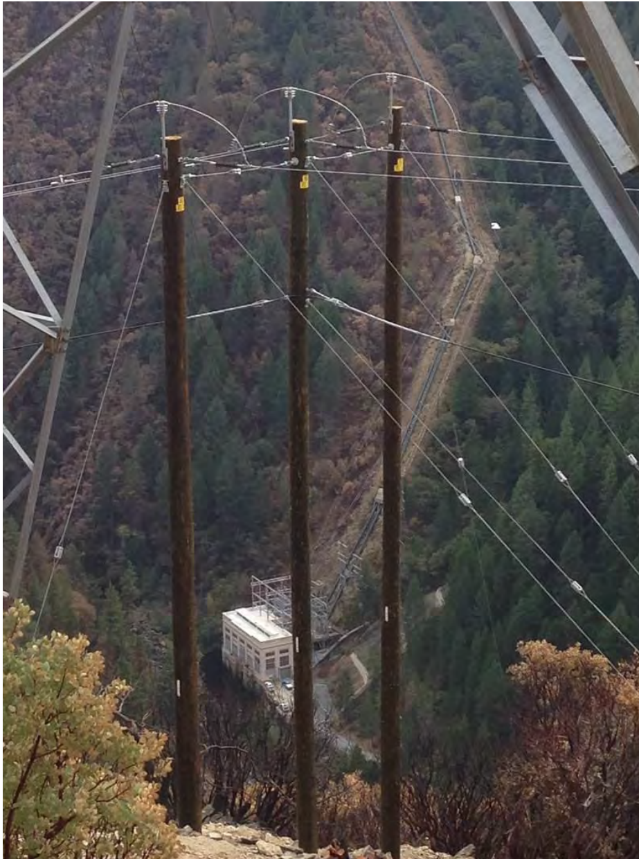
Photo 3. Poles from the rebuilt Brush Creek Tap Line showing APLIC-compliant design.
