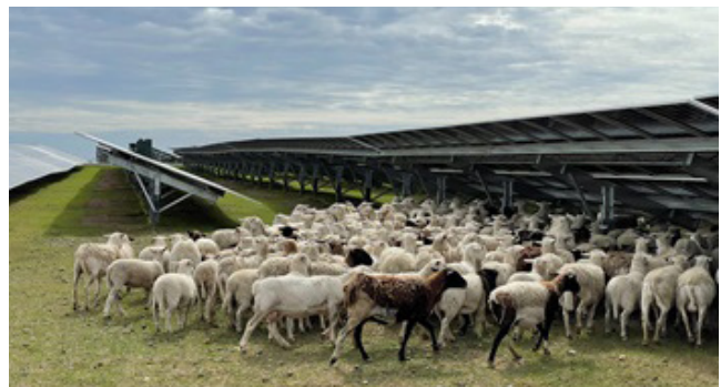
Sheep grazing around PV panels on site.
