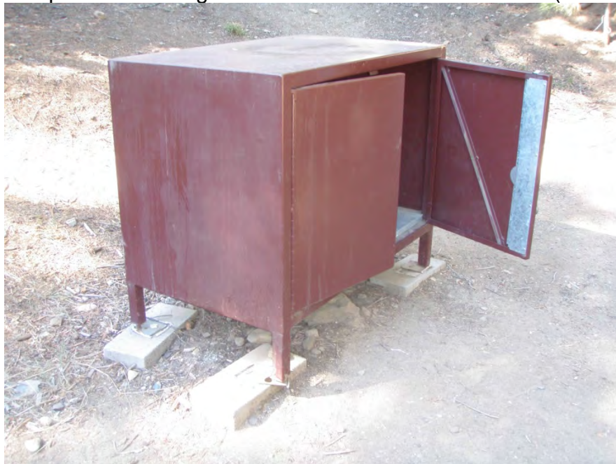
Photo 9. Bear-proof locker in good condition but with an unstable (off-center) footing.
