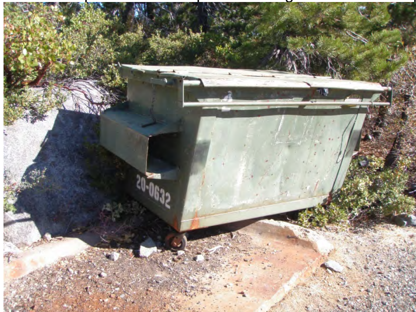
Photo 5. Bear-proof trash receptacle misaligned on concrete pad.
