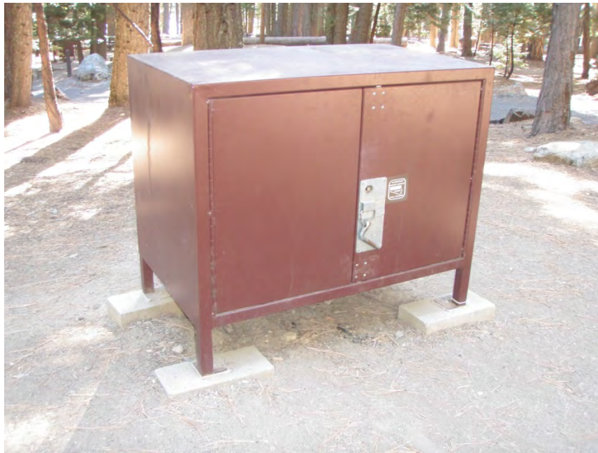
Photo 6. Bear-proof locker in good condition with concrete footings.
