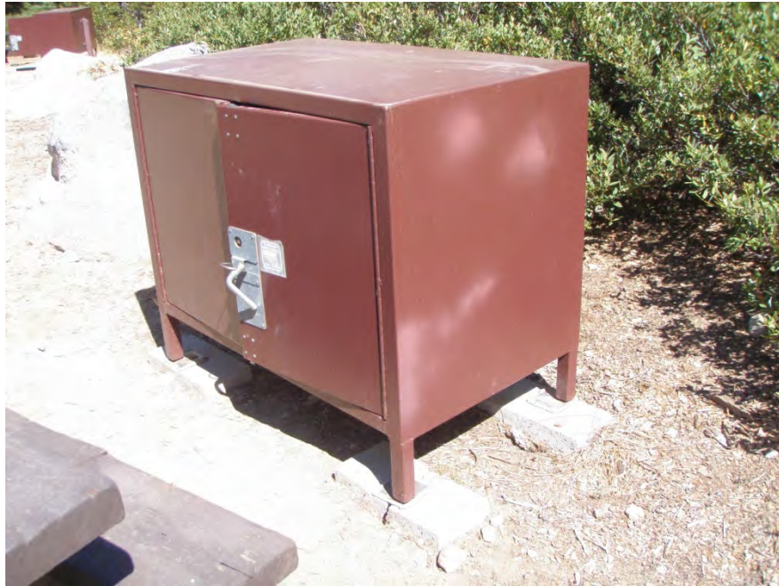
Photo 8. Bear-proof locker in good condition but with an unstable (cracked) footing.
