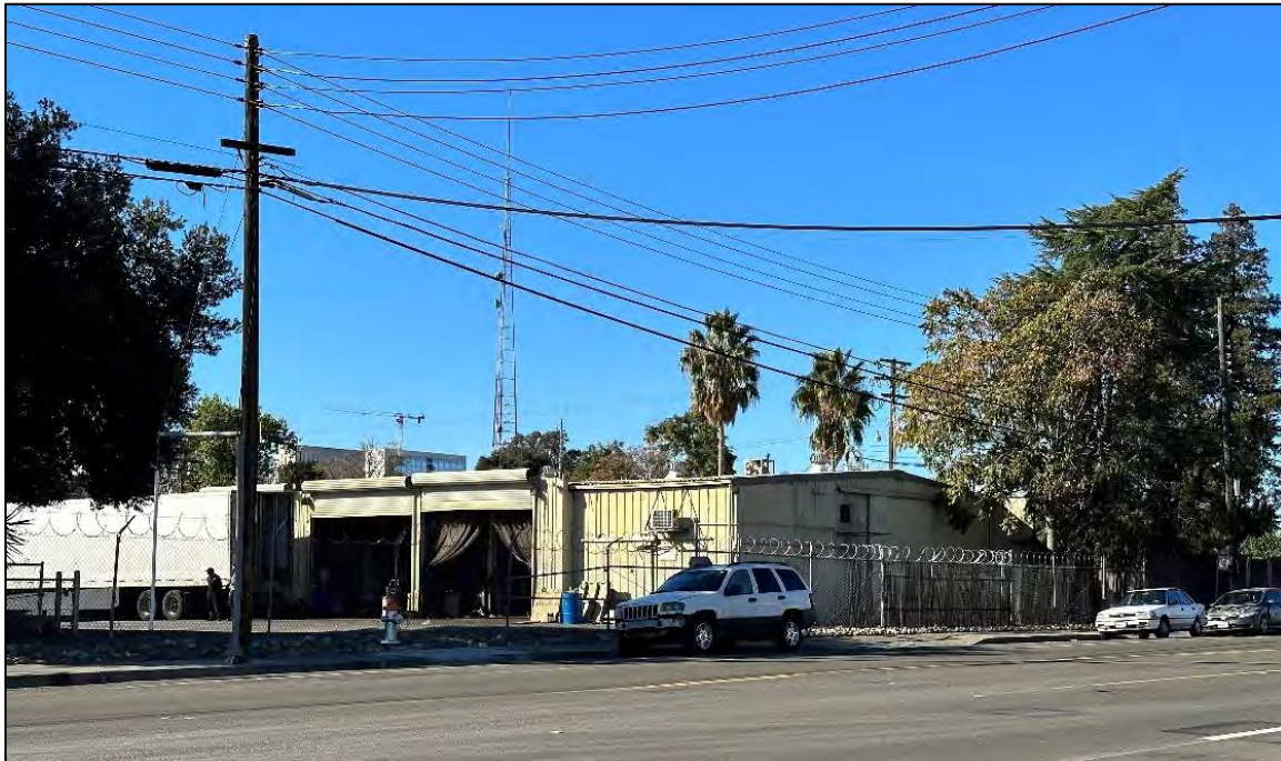
Photograph 4: 1226-1270 North B Street as viewed from North B Street, camera facing southwest, November 10, 2022
