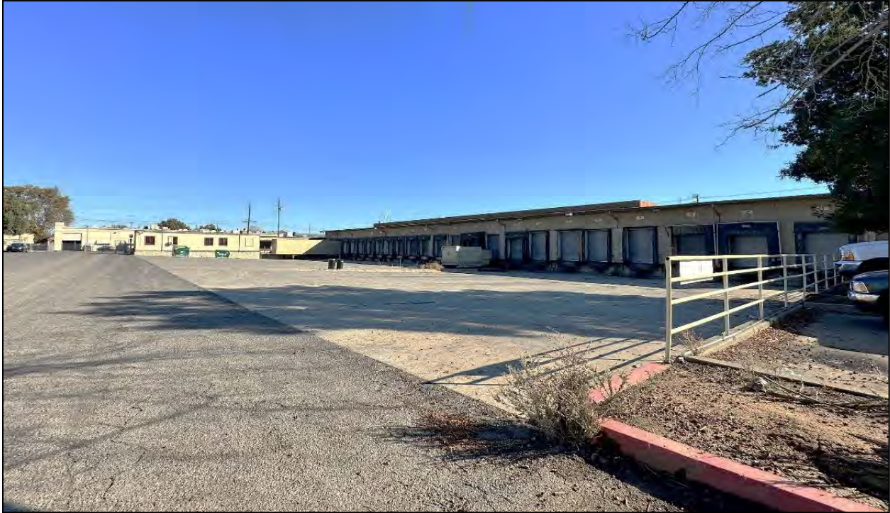
Photograph 3: West elevation of warehouse with 22 bays along the loading dock with slanted pavement, camera facing northeast, November 10, 2022.
