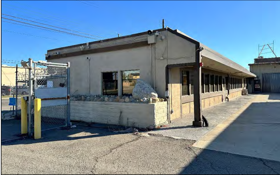
Photograph 2: Office building, camera facing northeast, November 10, 2022.
