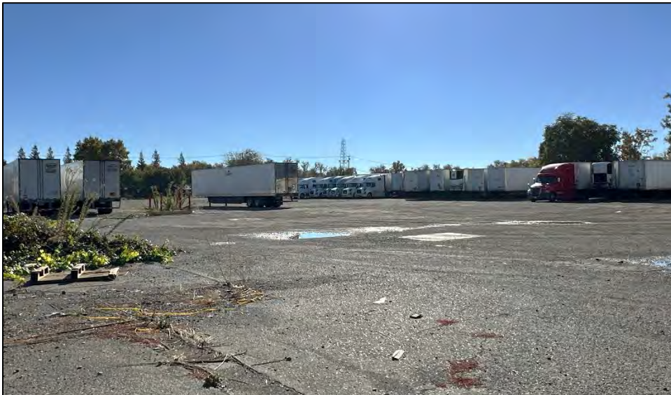
Photograph 7: Large parking lot area on APN 002-0041-083 sited south of the warehouse, camera facing southeast, November 10, 2022.
