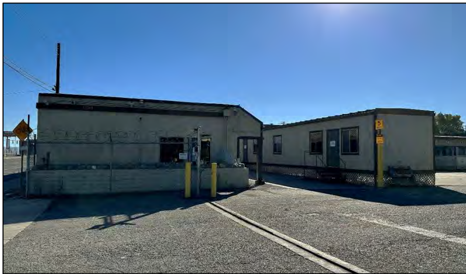
Photograph 3: Office building and parallel modular building, camera facing east, November 10, 2022.
