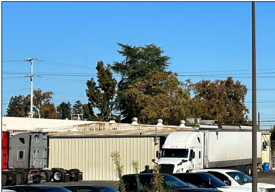
Photograph 3: South end of building with shed roof metal clad addition, camera facing northwest, November 10, 2022.
