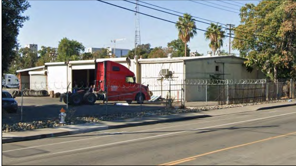
Photograph 2: East elevation of building with overhead roll-up doors, camera facing southwest, (Google Streetview October 2022).
