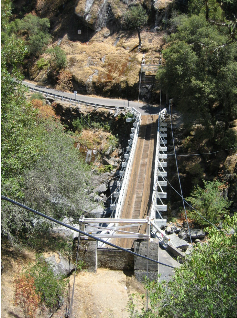
Figure 4.4-2. Mosquito Road Bridge crossing of the SFAR.
