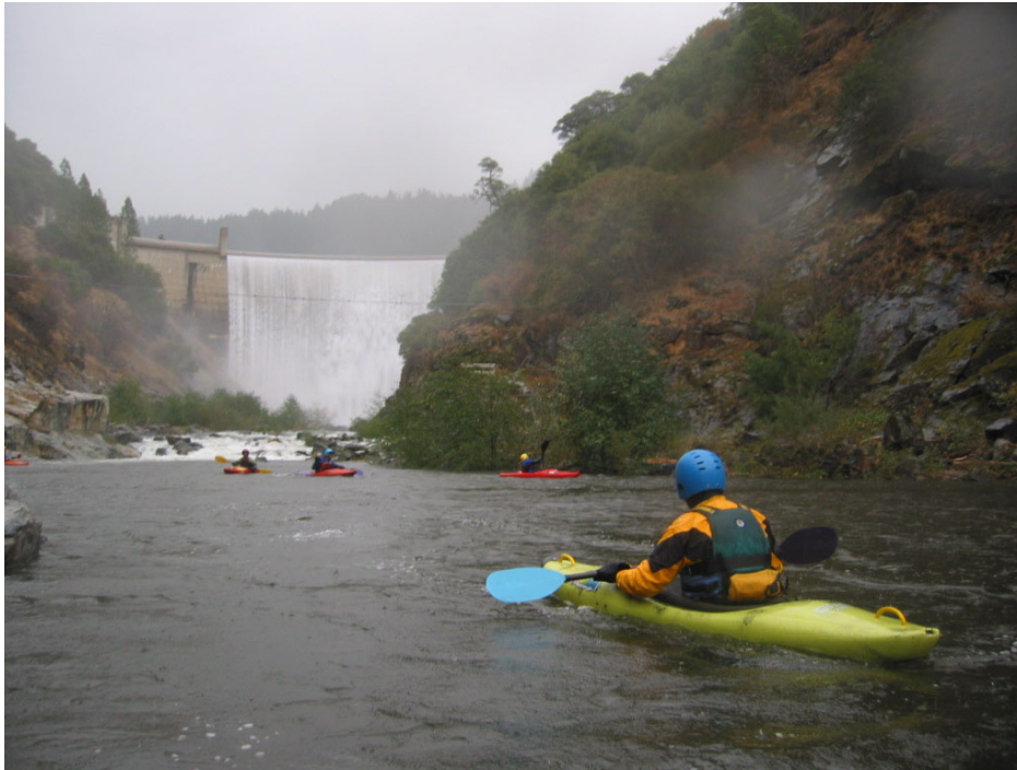
Figure 3.3-1 Slab Creek Dam Spilling during flow study.
