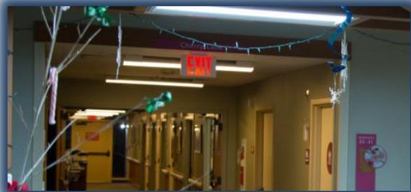
**Figure 16:** The new LED hallway lights significantly reduced the amount of glare and use 70% less energy than the fluorescent fixtures they replaced.
