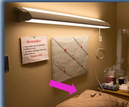
**Figure 18:** The push button switches for the LED overhead bed lights were too similar to the call light buttons.
