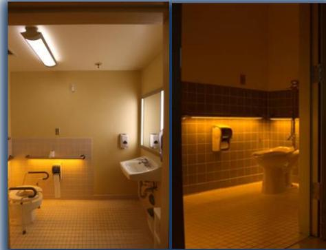
**Figure 6:** New handrails include integrated amber LEDs controlled via motion sensors.
