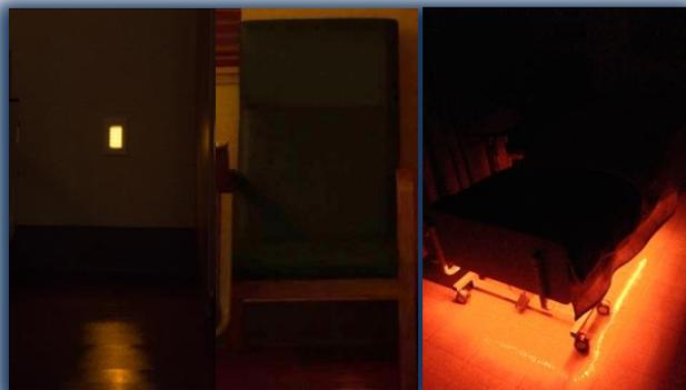
**Figure 17:** The wall-mounted LED nightlights (left side) did not work well because were often covered by chairs and other items. The LED lights mounted under the beds (right side) were much more effective.
