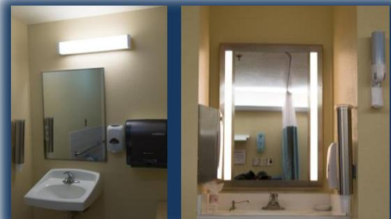
**Figure 5:** The original vanity lights produced a lot of glare (left side). The Project Team replaced these fixtures with dimmable, illuminated LED mirrors (shown on right).
