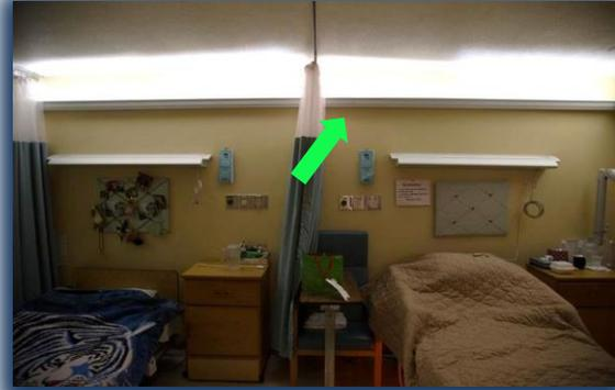
**Figure 3:** Tunable-white LED cove lights were installed in plastic gutters to shield residents from potential glare.
