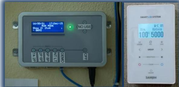
**Figure 15:** The controls for the LED cove lights (left) were much too complicated. The controls for the rest of the lighting were more intuitive yet lacked clear instructions.
