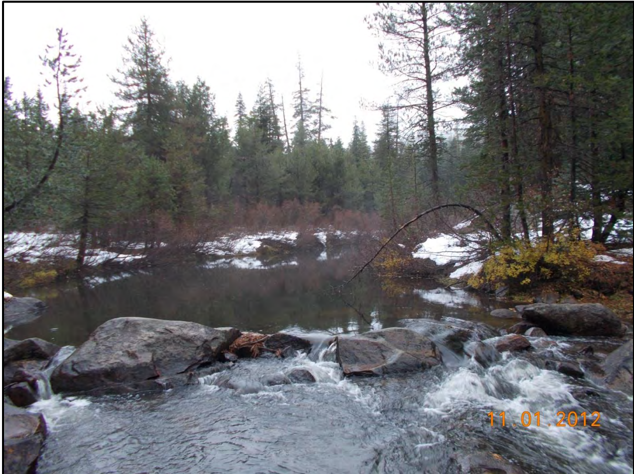
Figure A-1. Upstream View of the Boulder Lag Deposit that Provides Hydraulic Control Upstream into Gerle Meadow.
