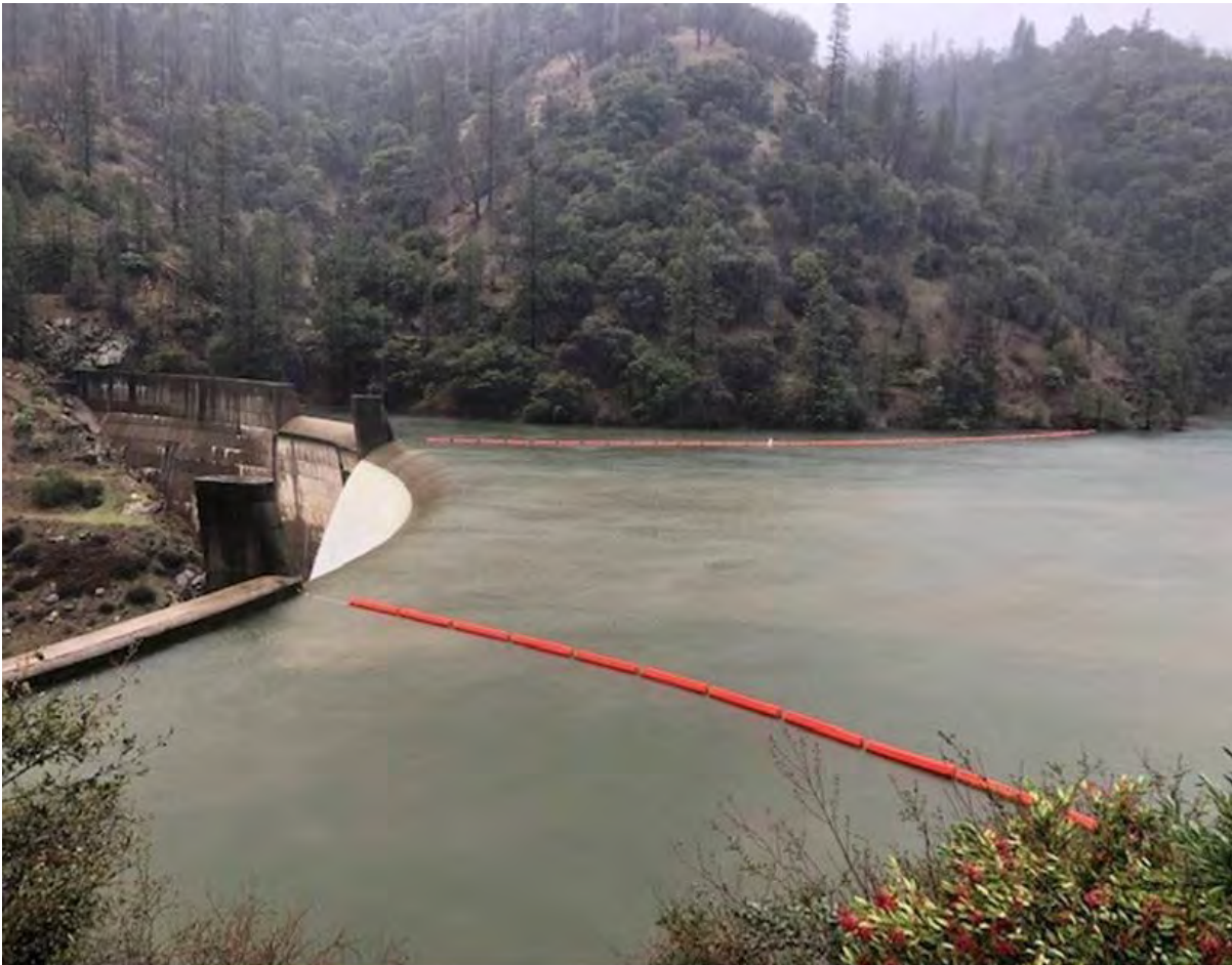
Figure 11-1. Log boom reconfiguration at Slab Creek Dam allowing large woody debris to move downstream.
