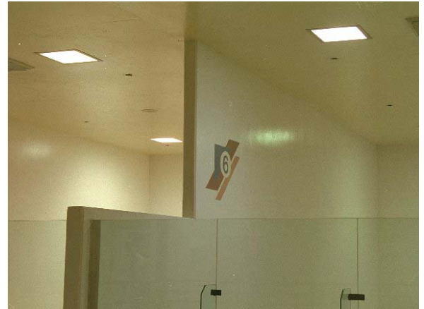
Photos of a racquetball court. Note how much brighter the court is after the T5HO system retrofit (shown on the left side).
