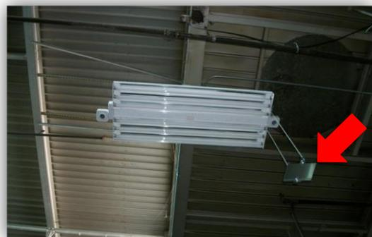
Figure 1-1: Steel plates installed below the sensor
