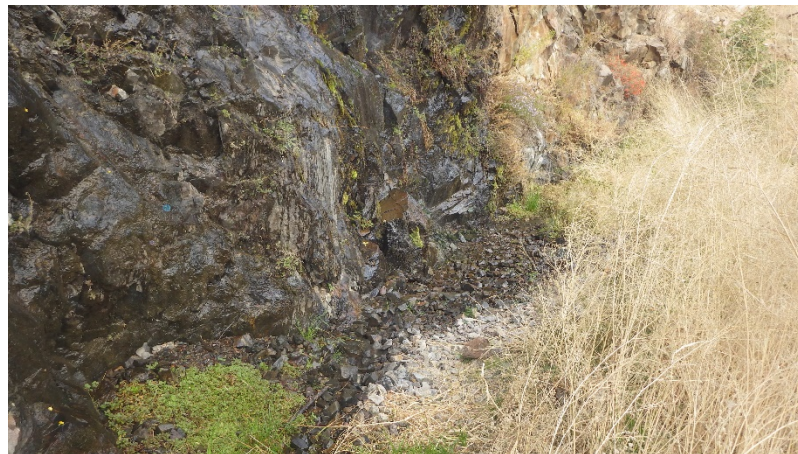
Seep on October 2, 2018
