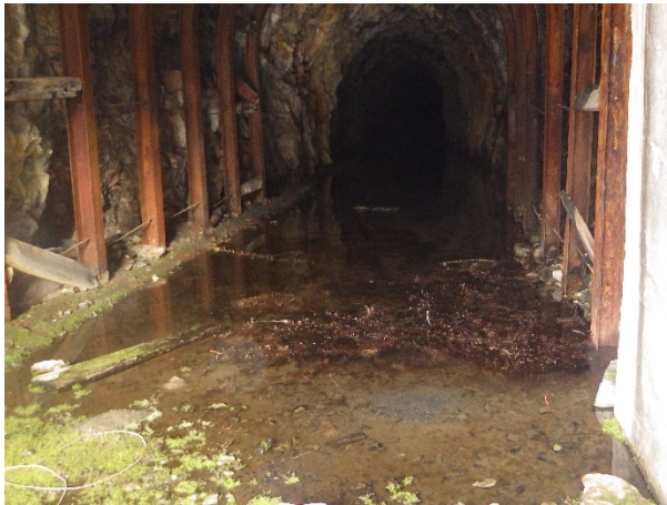
Camino Adit on October 2, 2018
