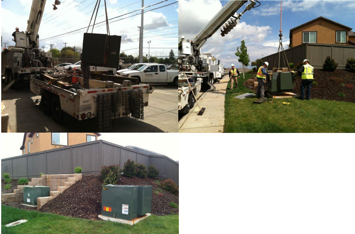
Figure 2. Collage of CES Installation
