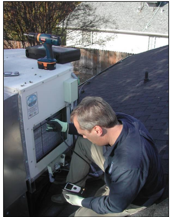
Figure 11: During 2009, new HMXs were installed in the Coolerados. During subsequent inspections, no visible mold was found.
