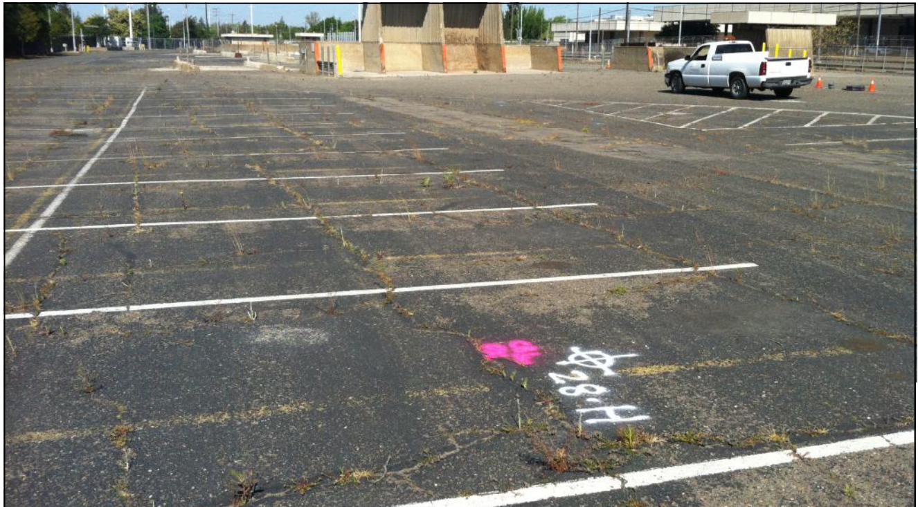
Image 36: KA-28-H is located southeast of the South Corporation Yard
