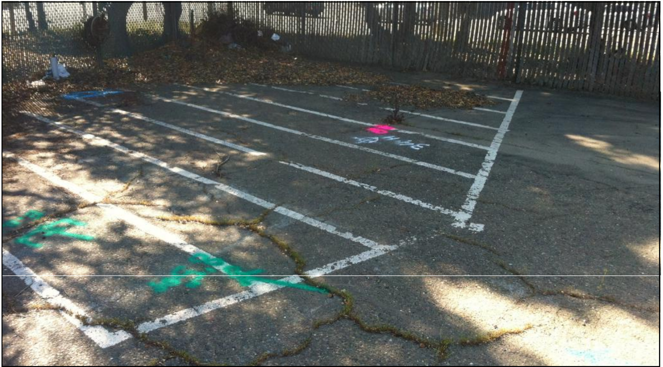
Image 35: KA-34-H is located southeast of the South Corporation Yard
