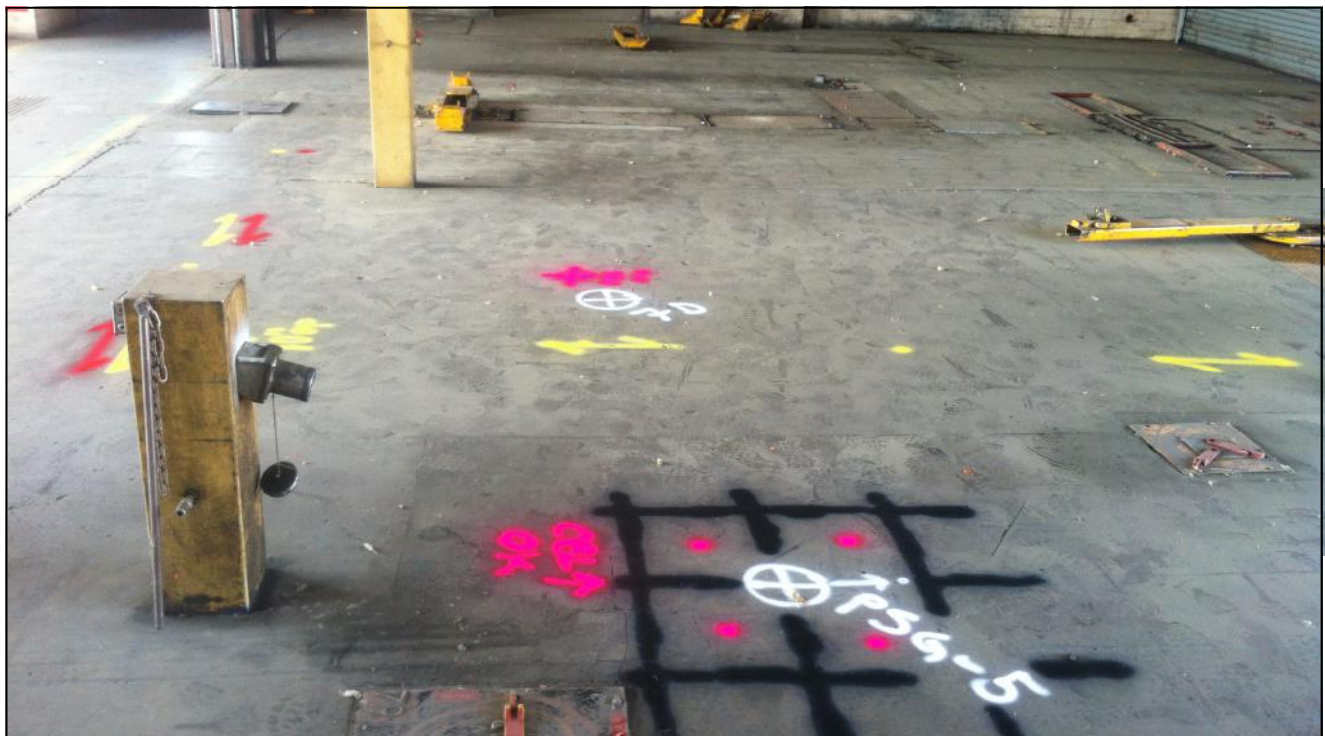
Image 8: PSG-5, KA-7-D, and KA-2-S are located inside of the Garage Building
