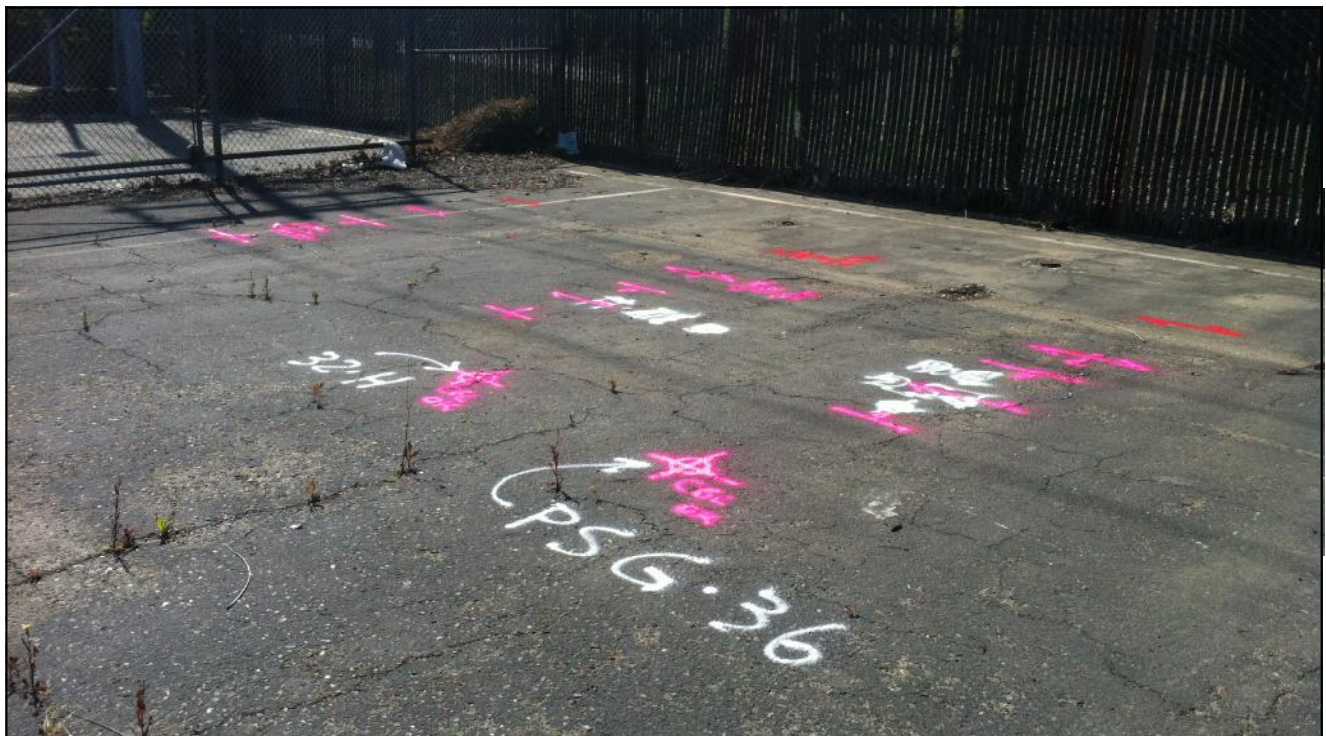
Image 48: PSG-36 and KA-32-H are located southwest of the South Corporation yard
