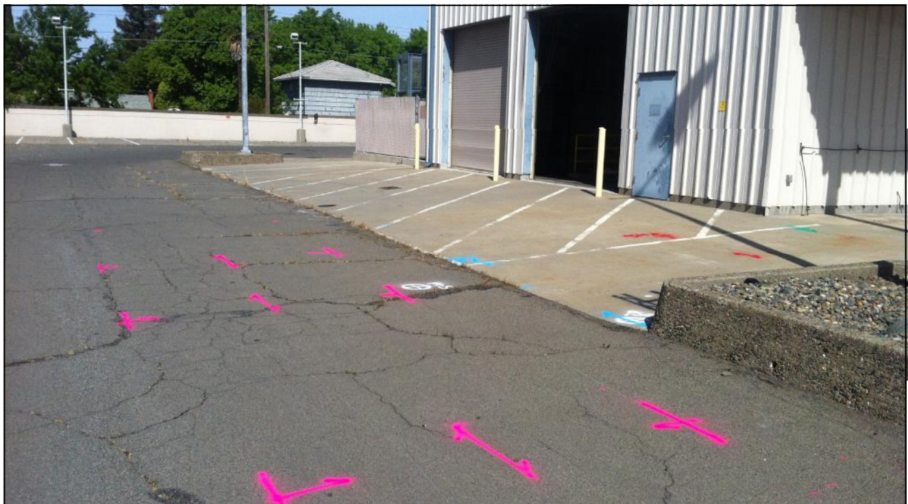
Image 20: PSG-18 and KA-14-S are located southeast of the Hazardous Material Building
