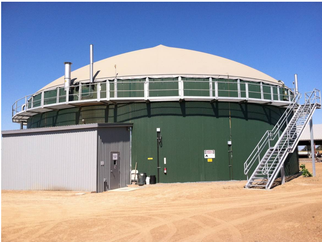
Figure 4. 1-million gallon tank digester at New Hope Dairy.
