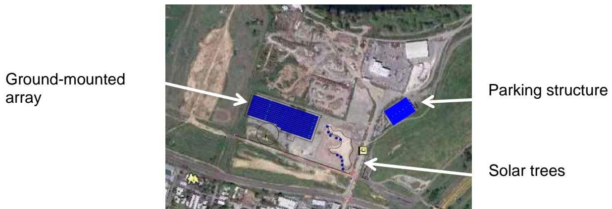
Figure 3. Aerial image of the three solar photovoltaic systems
