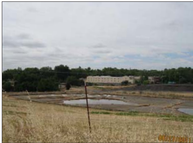
PHOTO 7: View southeast of concrete lined detention basin on the southwest side of the study area.
