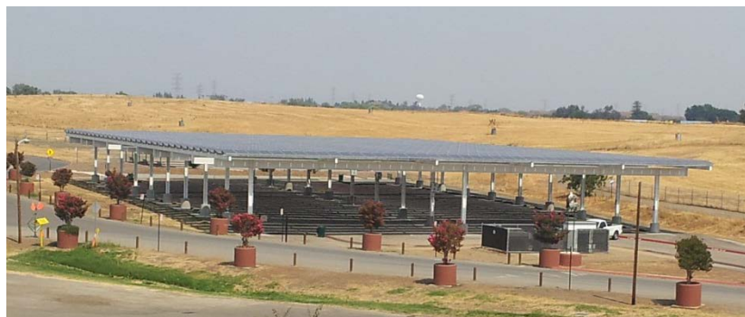
Figure 4. Photograph of the parking structure
