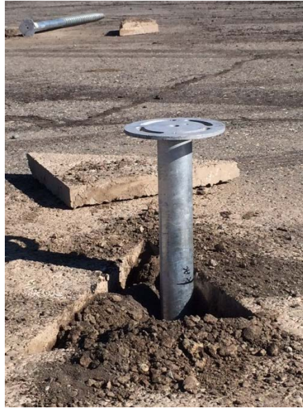
Figure 2. Earth screw foundation
