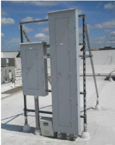
*Power recorder mounted next to electrical panel on roof.*
