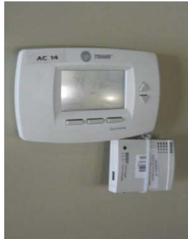
*Hobo temperature logger attached to thermostat.*
