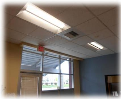
Figure 19: New LED lighting fixtures
