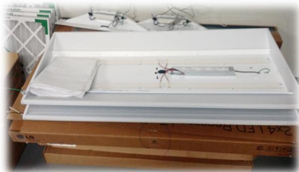
Figure 10: LED troffer disassembly to install wireless chip.
