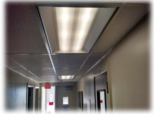
Figure 8: New LG LED lighting fixtures
