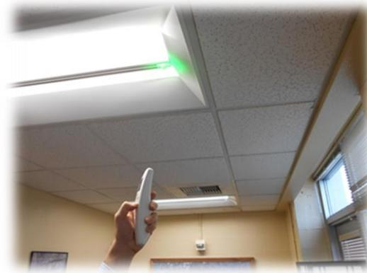
**Figure 21:** Installers said the commissioning was frustrating and time consuming, due to the slow speed of the remote control and the lack of an instruction manual.
