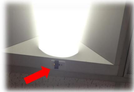
**Figure 14:** Some users were frustrated with the limitations of the remote control and resorted to using tape to cover the sensor to keep fixture in the “low output” mode.
