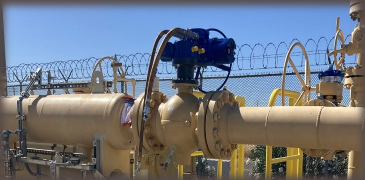
Valve Actuator Electrification
