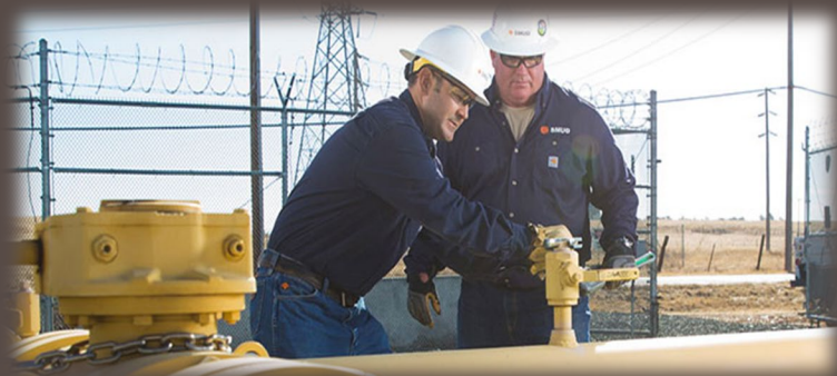
Immediate Leak Repair
