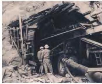
Workers check the progress of a drilling rig during the first construction stages of the Jaybird Tunnel in September 1958. The drilling lasted approximately 2 years as the tunnel grew to nearly 4 miles.
