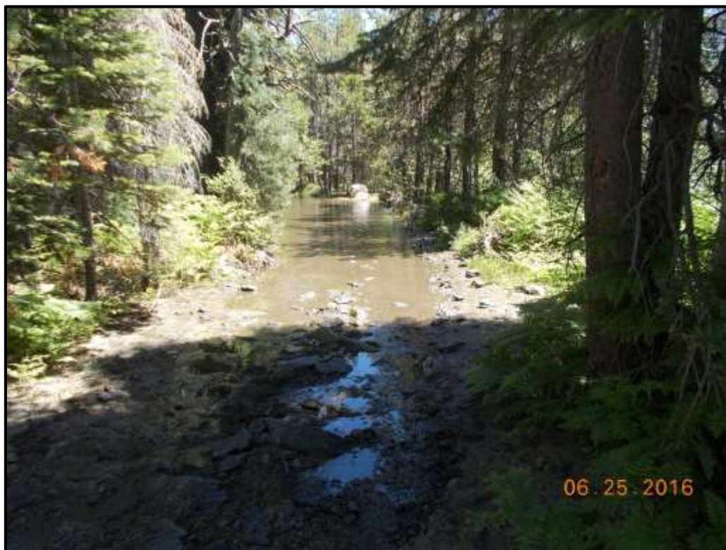
Figure 9. Flooding of county road into Wentworth Springs Campground, at about 375 cfs
