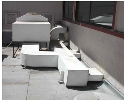
**Figure 7:** A poorly installed indirect-direct evaporative cooling system. The ductwork is far too restrictive to deliver the airflow needed to meet the cooling requirements of this classroom.<sup>6</sup>
