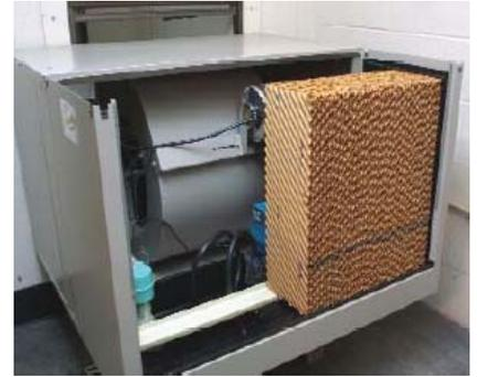
Figure 3: Direct evaporative cooler with rigid sheet pads<sup>5</sup>
