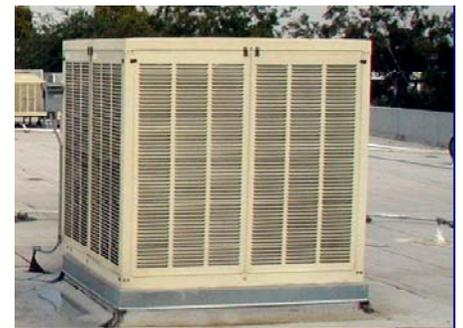
Figure 2: Fiber-pad direct evaporative cooler with aspen pads
