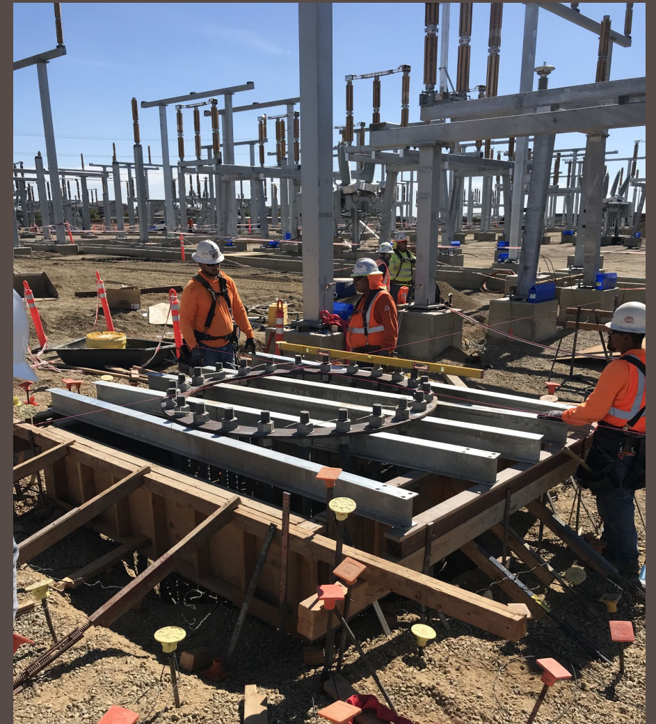
Station E 115kV Tower Construction
