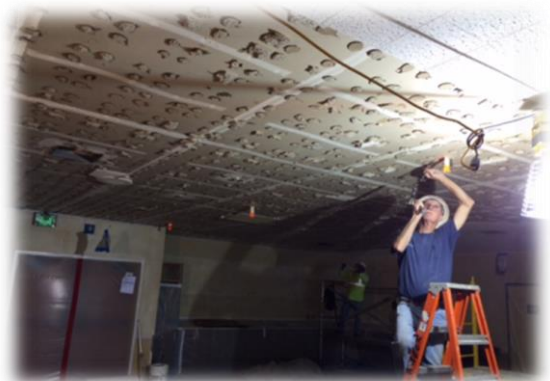
Figure 2: Removal of ceiling tiles was a daunting task when it was found they were glued to the ceiling and the old glue had to be chiseled off.
