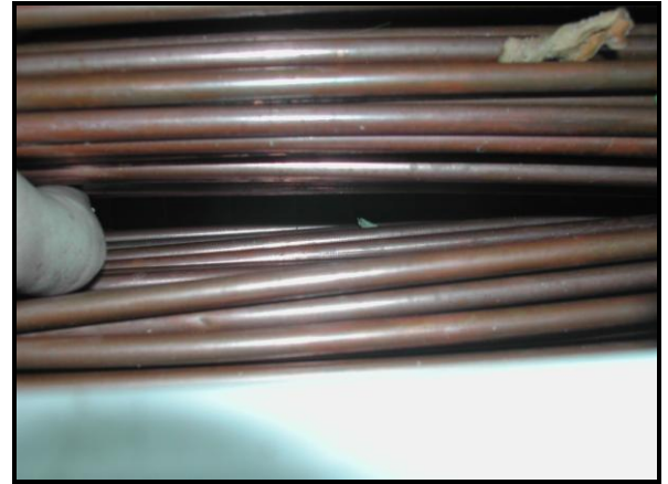
Figure 4: AquaChill's condenser coil consists of a bundle of flexible tubes that are suspended above the water basin. If hard water scale forms on the condenser tubes, it is dislodged by the expansion, contraction and vibration associated with normal operation of the unit.
