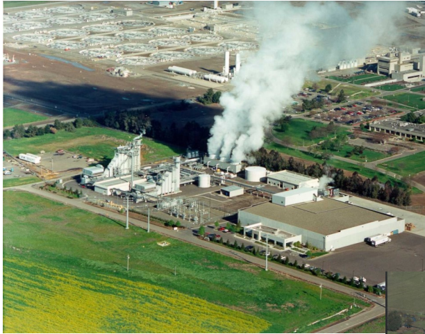
Carson Power Plant
