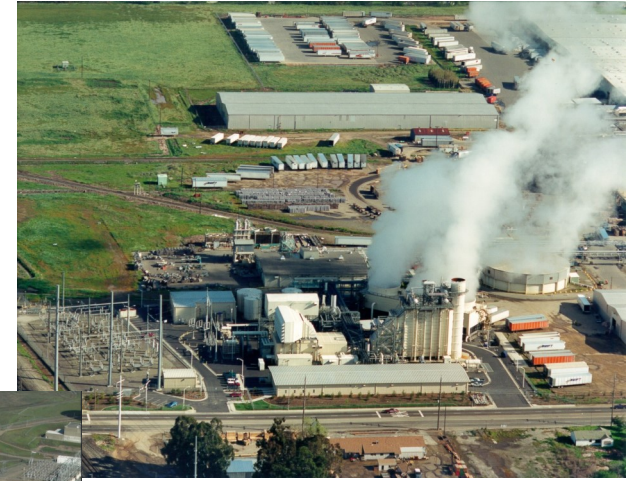
Campbell Power Plant
