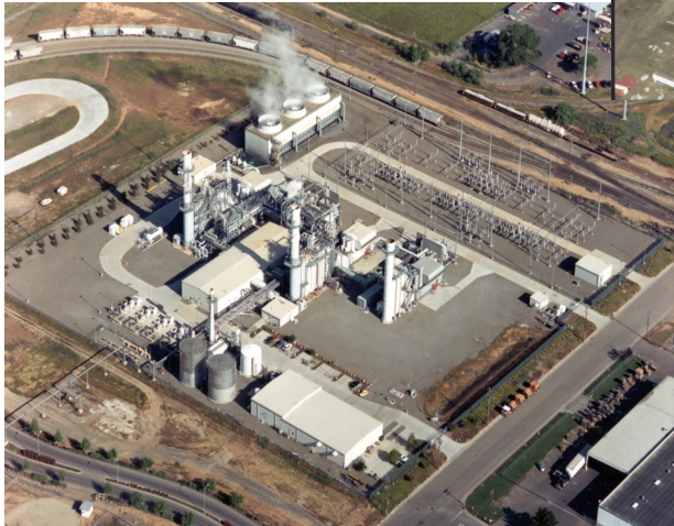
Procter & Gamble Power Plant
