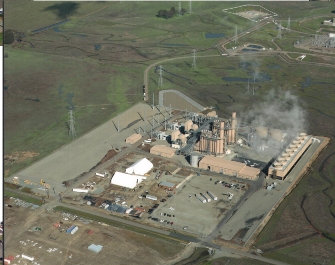
Cosumnes Power Plant
