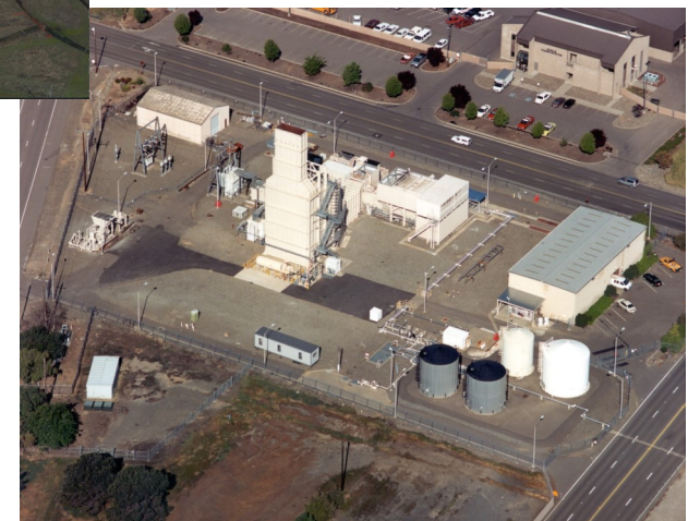
McClellan Power Plant
