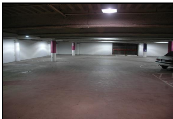
Figure 4: photos of the Sacramento City parking garage after the LED retrofit.
