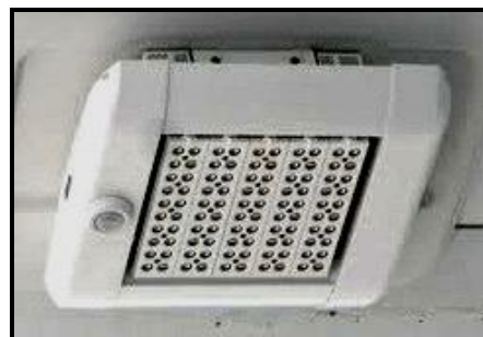
Figure 5: the LED fixtures at the City parking garage included integrated motion sensors similar to this one.
