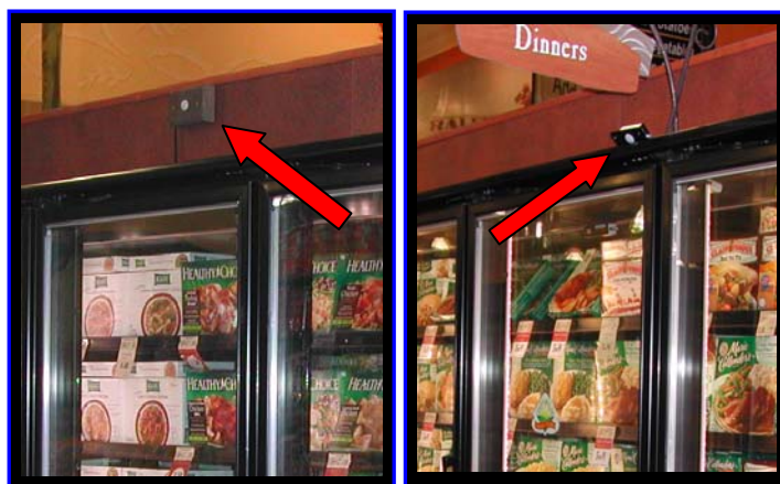
Figure 8: The prototype sensor (left) was mounted to a decorative façade above the freezer case. The final version of the sensor (right) was mounted directly to the frame of the freezer case.
