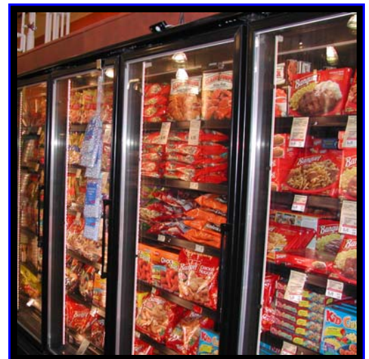
Figure 17: The new LED fixtures provide very even illumination for all of the freezer cases at this store while minimizing glare.
