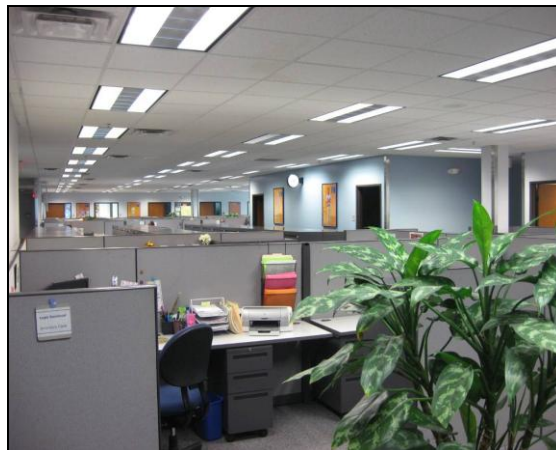
Figure 2: the original fluorescent lighting system
