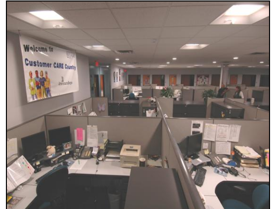
Figure 10: Although the new lighting system provided excellent illumination on desk top surfaces, it created somewhat of a “cave” effect in some areas of the office
